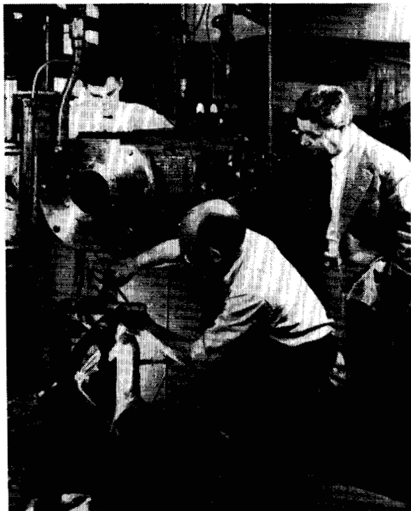
Fig. 10. MIT molecular beam apparatus, 1946. J. R. Zacharias watches John McClean, one of his two mechanical technicians, sweat together the apparatus of Fig. 5. In background is student Darragh Nagle. (Photo courtesy of the MIT Museum.)
